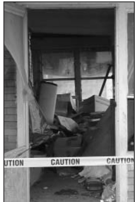
The inside of one our work-study houses before demolition
