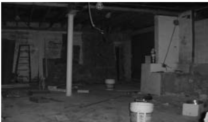
The kitchen's new pantry area under construction
