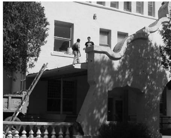
Michael Hunsberger, Construction Coordinator and student begin demo work
