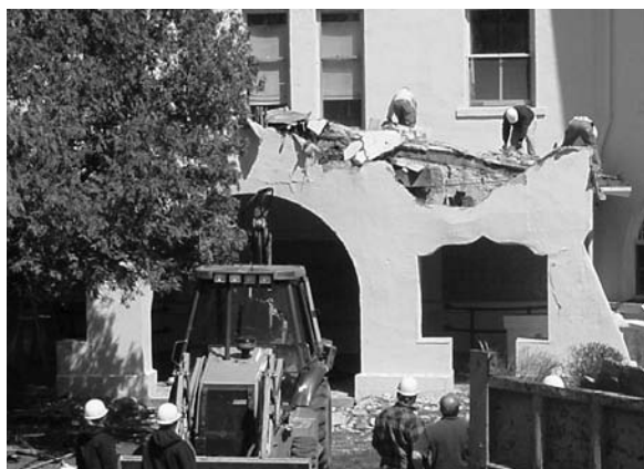
Demolition of the old porch portico
